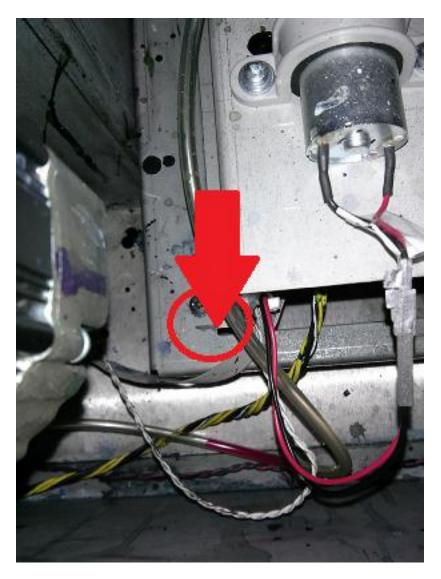
**2.1** Once the old maintenance station is removed, measure the position of the marks then use these measurements to draw the same marks in the same position on the new maintenance station.
